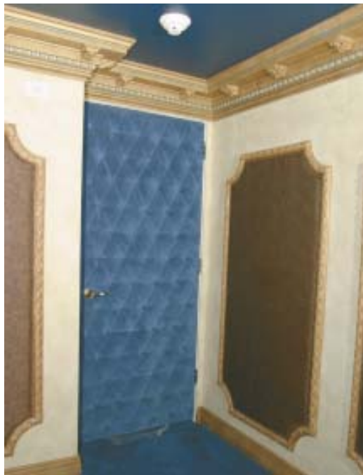
Figure 3. Theaters should contain a lot of sound-absorbing material such as carpeting, stuffed furniture, and heavy drapes. Upholstered panels have been added to the walls and door of this high-end dedicated theater.
