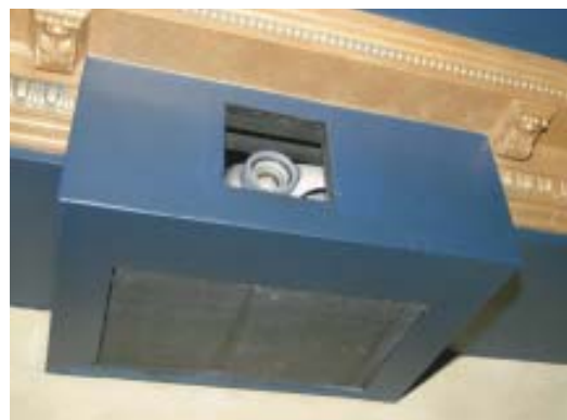
Figure 10. Projectors are noisy, so they're typically placed in soundproof enclosures. This unit projects through a piece of glass and can be serviced through the access panel below. The box is mechanically vented through the soffit to prevent the projector from overheating.
