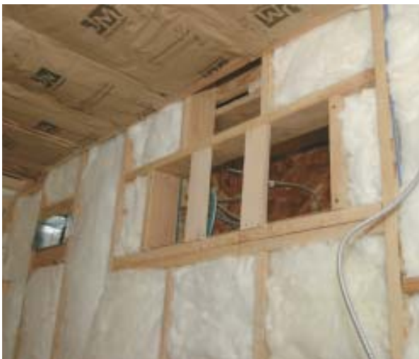
Figure 1. Soundproofing is important in the walls of a home theater. Here, a partition wall has been insulated to limit the amount of sound that reaches the adjoining room.
