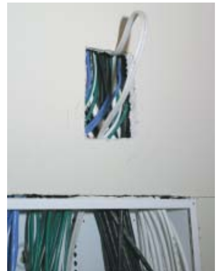
Figure 5. The electrician ran this Romex when no one was looking. It shouldn’t be in with the A/V cables and will cause interference if it’s not removed and brought in separately from below.
