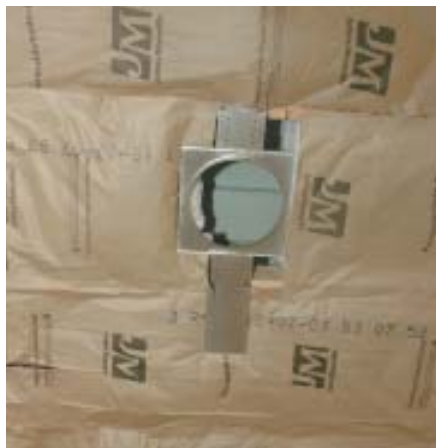
Figure 8. The rear speakers work equally well in the wall or ceiling. Everyone on site will have an opinion about where they look best, but check with the theater designer to find out where they'll sound best.
